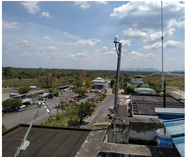
-GPS Timing Antenna External ,Outdoor w/Mounting Hardware, Low Loss Cable 20 M
