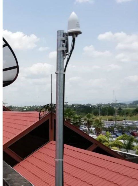
-GPS Timing Antenna External ,Outdoor w/Mounting Hardware, Low Loss Cable 20 M
