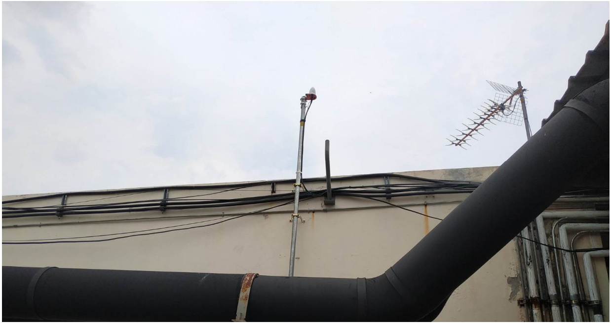
-GPS Timing Antenna External ,Outdoor w/Mounting Hardware, Low Loss Cable 20 M
