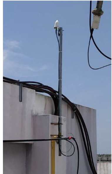
-GPS Timing Antenna External ,Outdoor w/Mounting Hardware, Low Loss Cable 20 M
